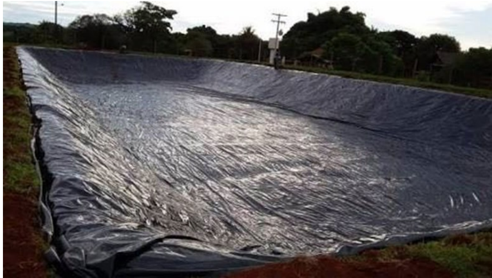
Figure 6: Rectangular tank coated with PVC geomembrane
