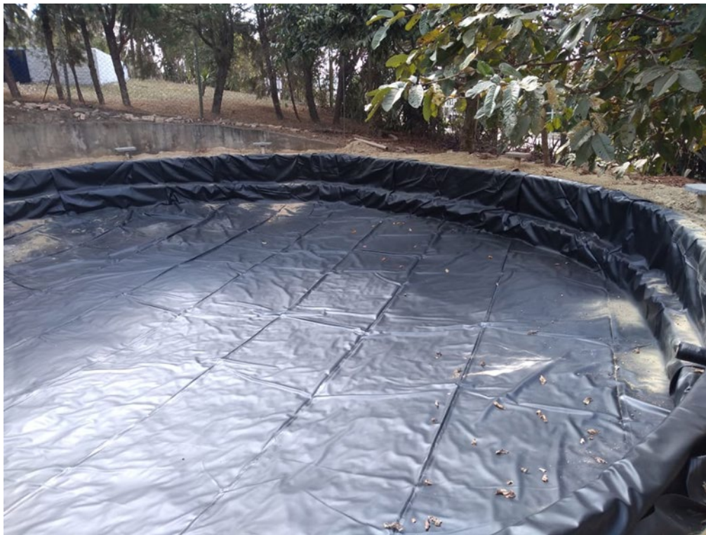
Figure 5: Circular tank coated with PVC geomembrane
